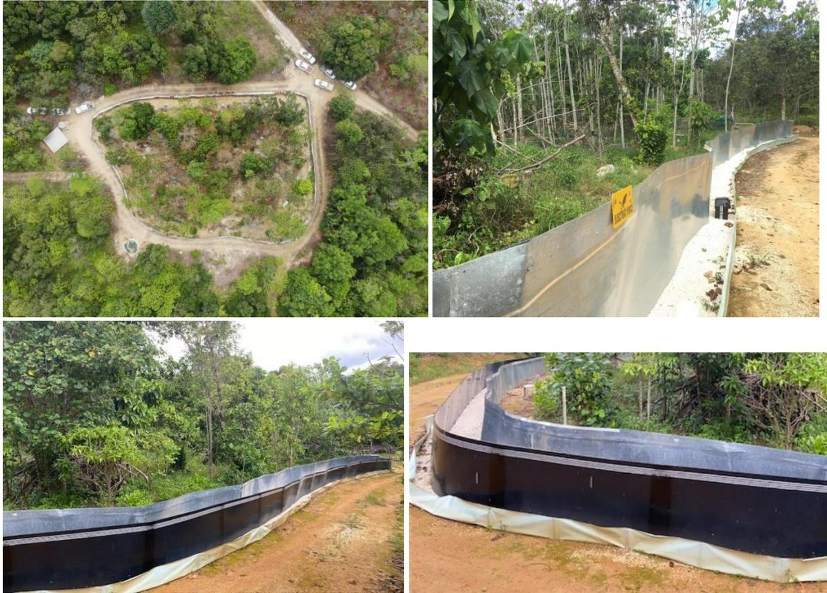
**Figure 1.** Photos of Circuits SRS: predator proof fence in 2018 (top left, right), and in 2022 after construction of second fence (bottom left, right)
