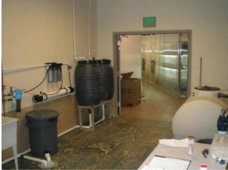
Figure 8. The building's water storage and central treatment station.
